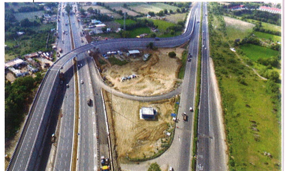
Dumad Interchange on Ahmedabad Vadodara Expressway (NE-1) & NH-8 Intersection Optimized by www.Imgix.com/interact.net
